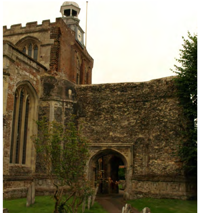
Plate 4.12 Current view of the north archway
